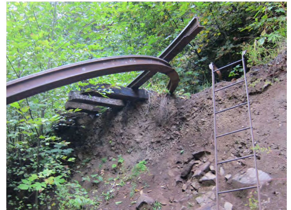
Damage at MP 806
