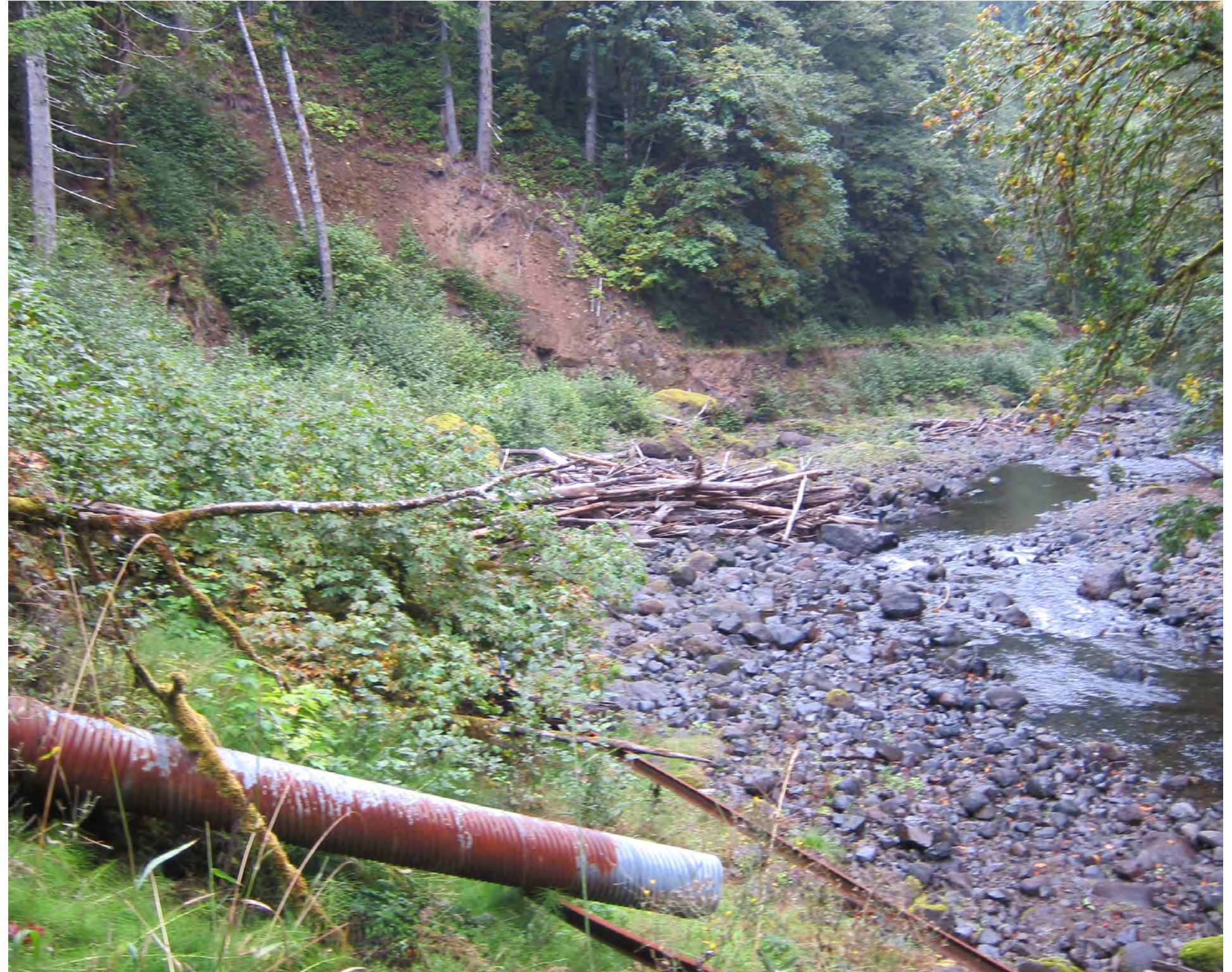
Salmonberry River bank erosion, Milepost 807
