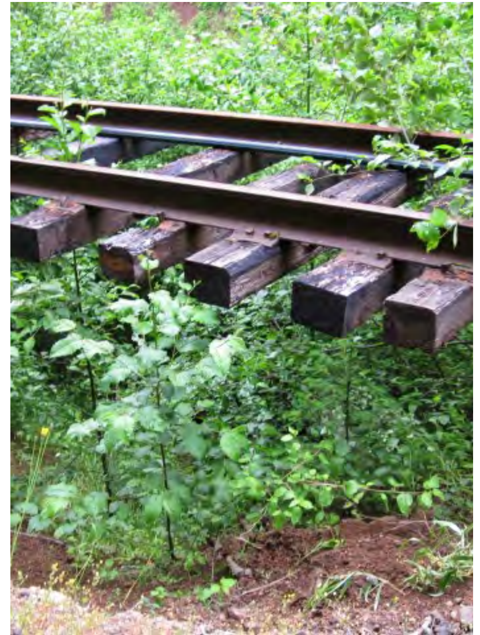
Rails and ties left hanging over damage point near Wolf Creek (Dan Kaufman)
