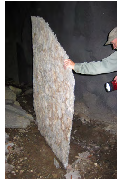
Gunite concrete fallen from ceiling of Walcott Tunnel
