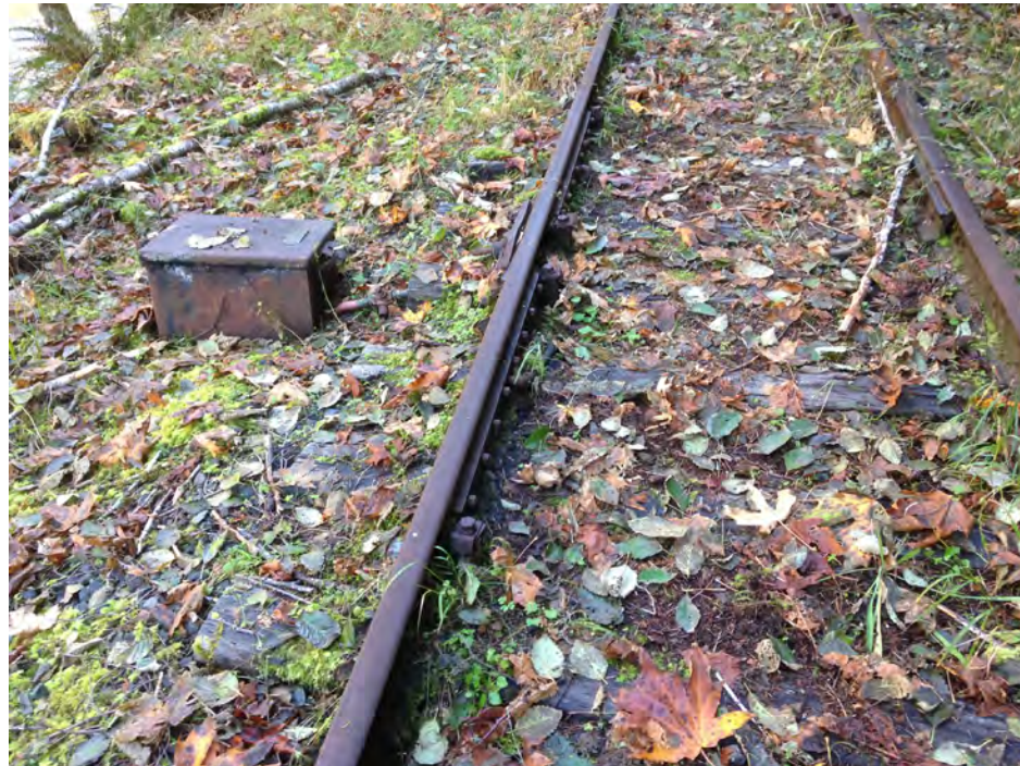
Oiler boxes next to RR tracks contain a petrochemical lubrication that must be secured to prevent leaks into the Salmonberry and Nehalem Rivers.
