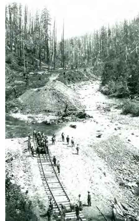
Rail Construction, Nehalem/Salmonberry Confluence, 1911 (Punk Rotten & Nasty, 2001)
