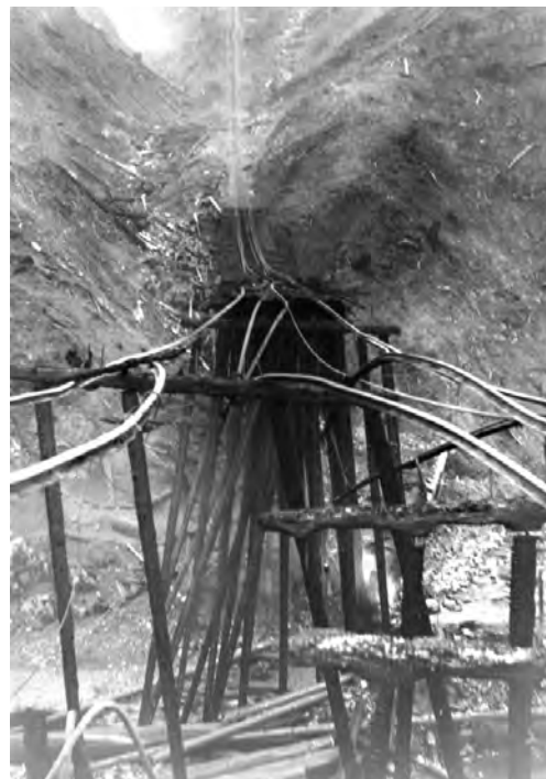
Base of the West Oregon Lumber Company incline near Belding following the October 1932 Cochran Fire. Trestle crossed N. Fork Salmonberry River at its confluence with the Main Fork.
