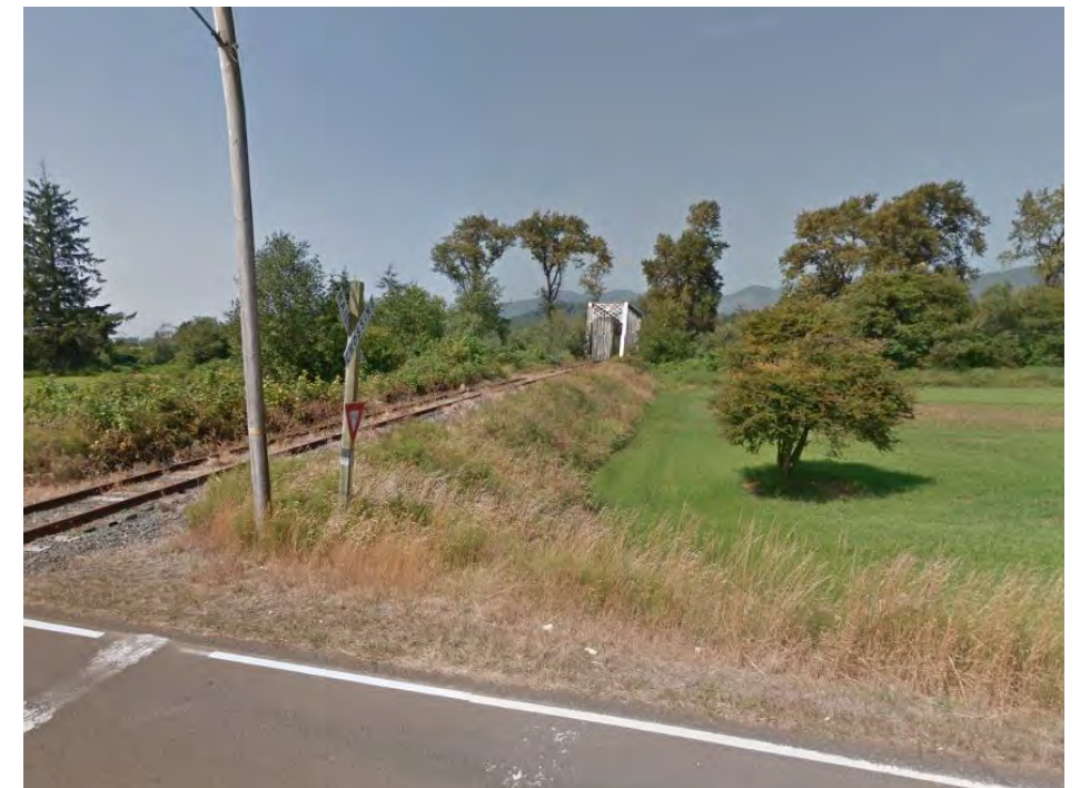
A typical embankment on the Coast, raising the line above dairy farms, wetlands and floodplains
