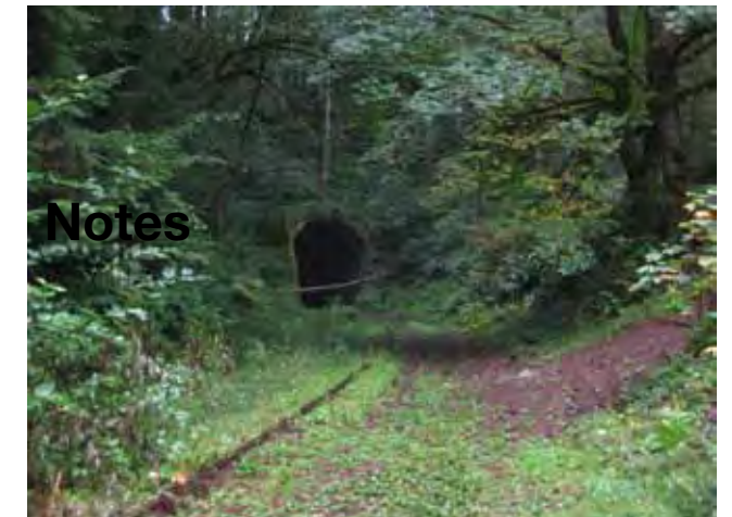
View east to Tunnel at Beaverslide
