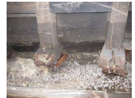
Damage to Walcott Tunnel structure
