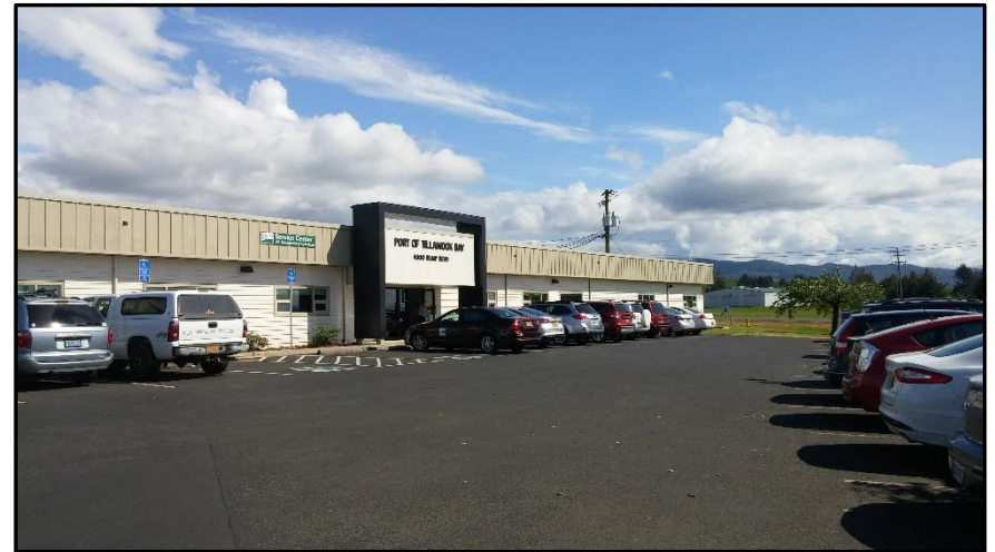
POTB Office Complex on the north side of POTB land.
